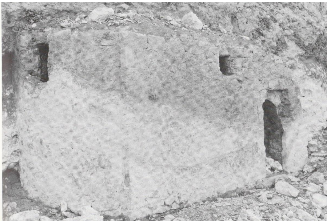
Plate 14: St Andrew Chapel, 1963 (photo probably by D Winfield in Bryer and Winfield 1985:plate 165a).
