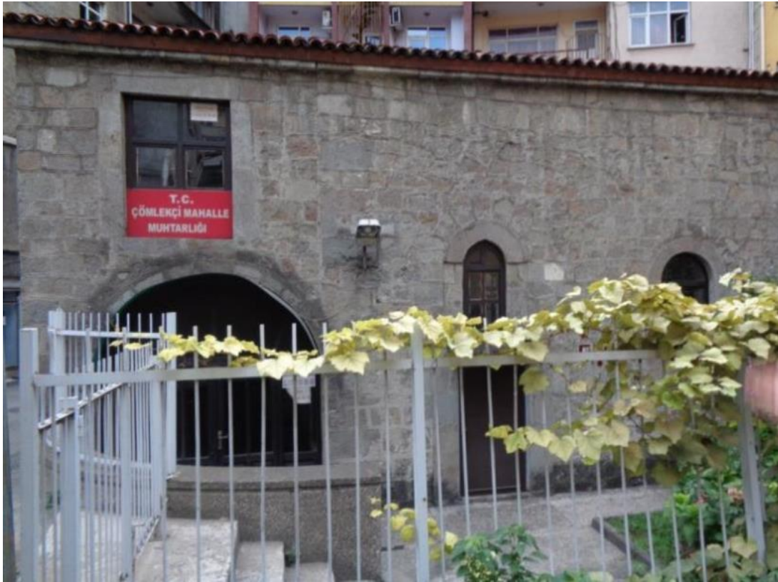
Plate 37: Former church, name unknown, the three apses are to the right of the photo—Çömlekçi district, Muhtarligi building (author's photo 2018).
